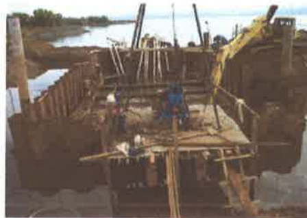
Figure 14. Excavation of Case 2 Project
